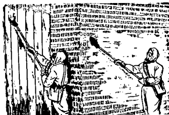
Decontamination of Walls with the Calcium Chloride Paste.
